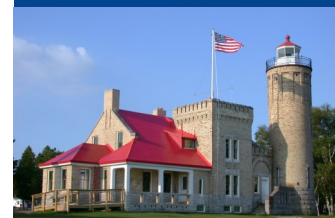
Mackinac Point Lighthouse
